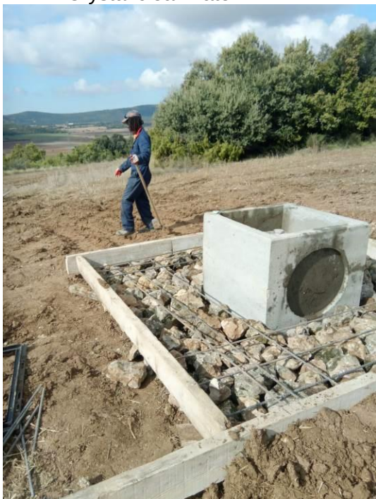
Formwork for floor slab
