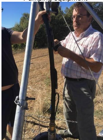
Installation of automatic sensors
