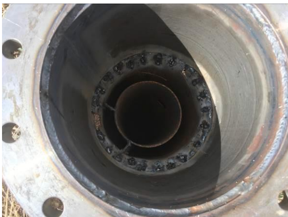
Inside of the well
