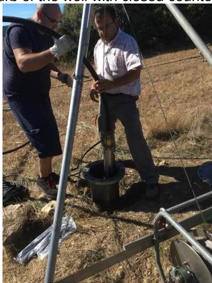
Insertion of pump in well
