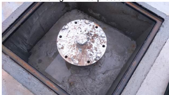
Borehole inside manhole
