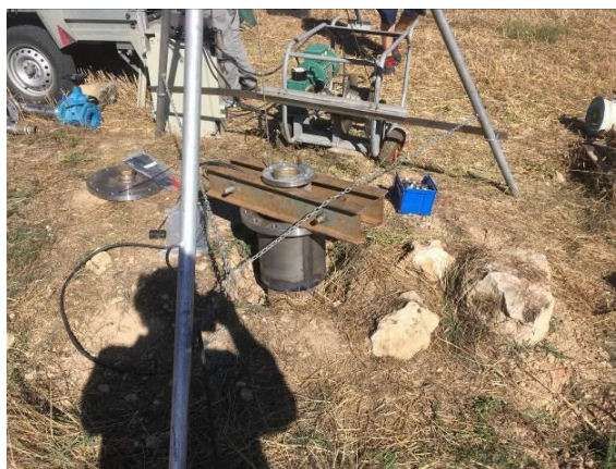
Installation supported on joists
