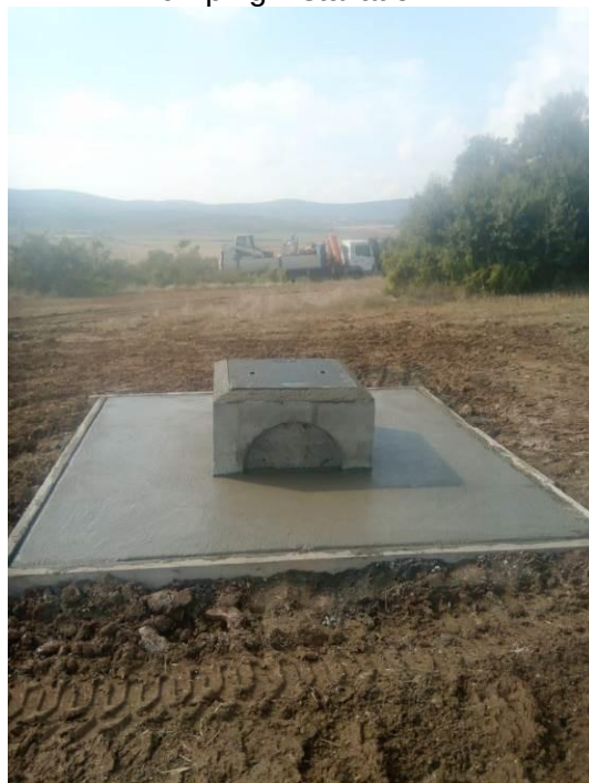
Building work to protect well
